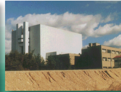
Super GE (Super Conductive Electric Generator)
