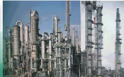
Chemical Plant (EG & NH 3 )
